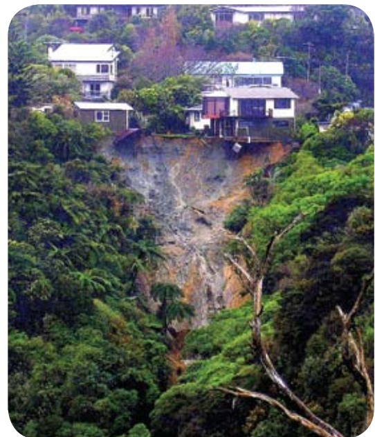
Large landslide in Kelson, Lower Hutt (2006).
